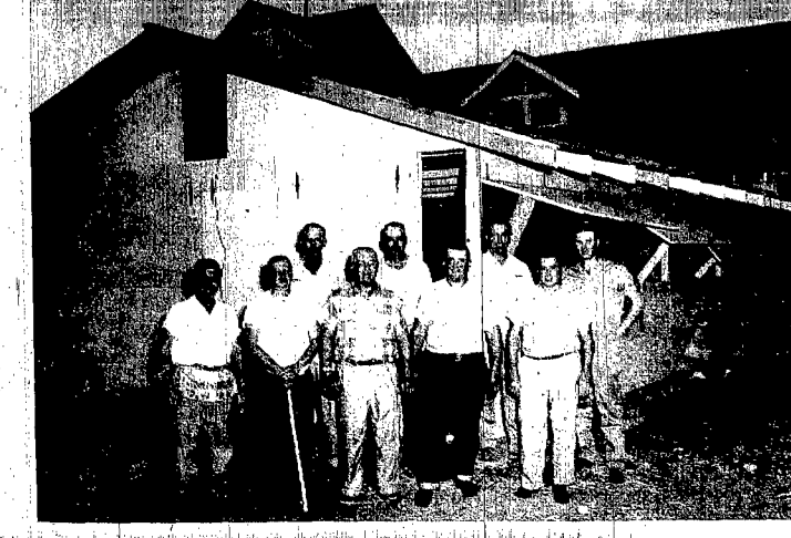
WORK IS NEARING COMPLETION on the earthen stand at the Wayne County fairgrounds. The stand is financed by a grant from Ak-Sar-Ben. These men and others have donated their labor to keep costs down. The stand will be operated by the St. Mary's church, who have donated much of the labor. The workers are: front row, Otto Botsford, foreman; Clate Sharer, Al Bahre, Jerry Pospisil and Joe Lowe. Rear - Ray Langemeier, John Lynch, Gib Shald and Ray Starman.
